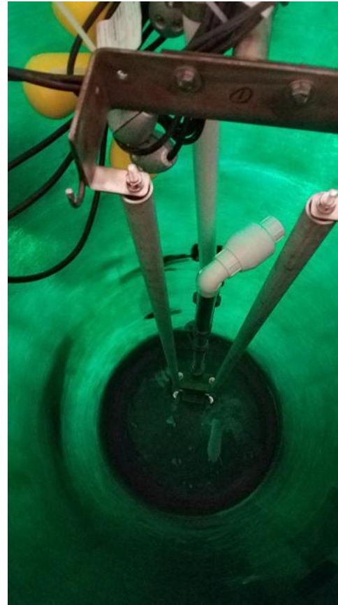
Top: Inside of a grinder pump basin; Right: easy access to grinder pump basin.
