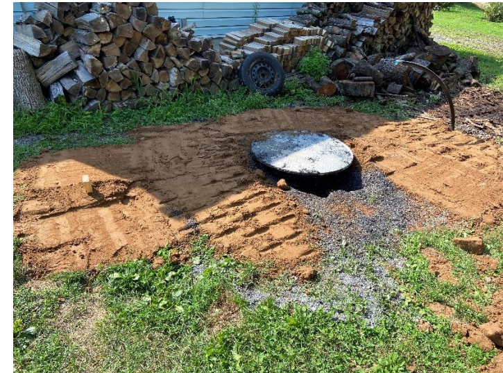
Installation of grinder pump system
